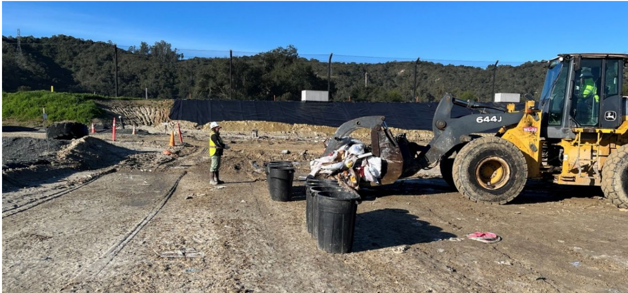
Figure 3-4 Loader Delivering Sample Material to the Staging Area
